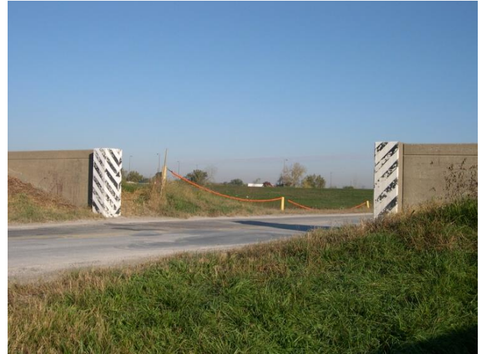
Figure 1: Closure Structure in Prairie du Pont
